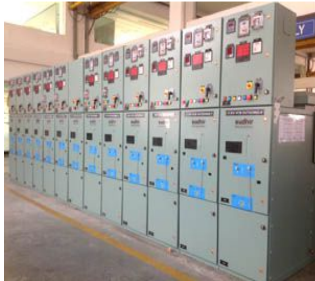
Pictorial representation of HT Panels
